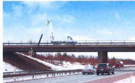
Ability to work below ground level (-3,3 meters)
